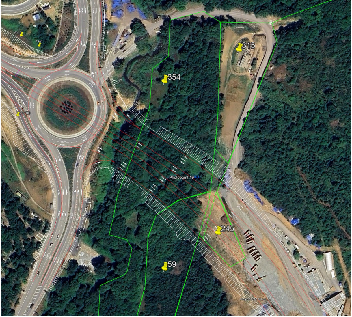
Figure 3 Parcel status of parcels 246 and 271 after land acquisition
